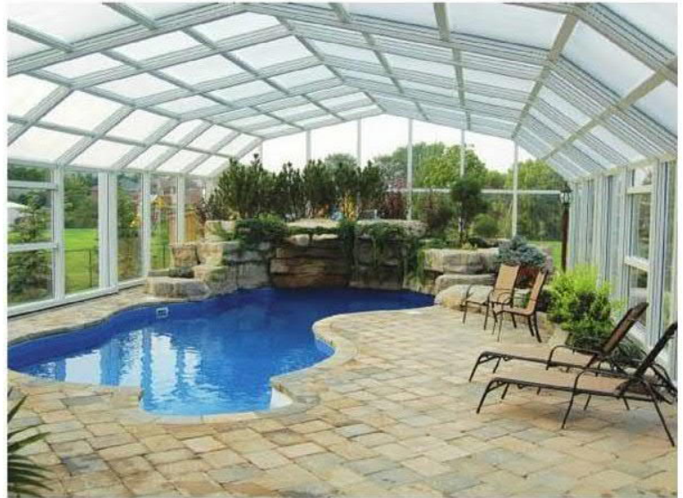
The size of an enclosure is primarily determined by its intended purpose and client preferences. For this home in Ontario, the enclosure was built to shelter the pool, patio and various landscaping features so they could be enjoyed year-round
